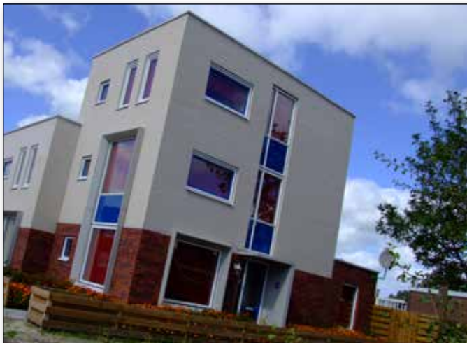
Lemmerweg-Oost, Sneek (NL), wastewater treatment for 32 houses realized in 2005
